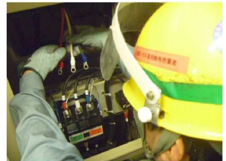
(直流き電盤内NFB2次側へ接続)
